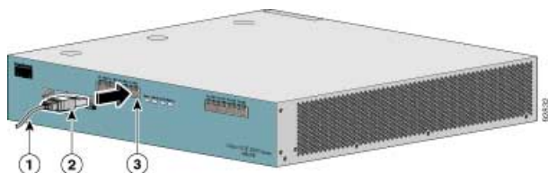
Figure 18: Cabling the FE Interface
